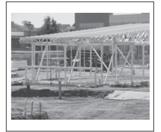
Construction of the new **Child Development Center** at City College is underway. The five low-profile buildings on Judson at Gennessee are being built using sustainable, green design. Building roofs, for example, will be covered with drought-resistant succulents that will provide insulation for the buildings.
